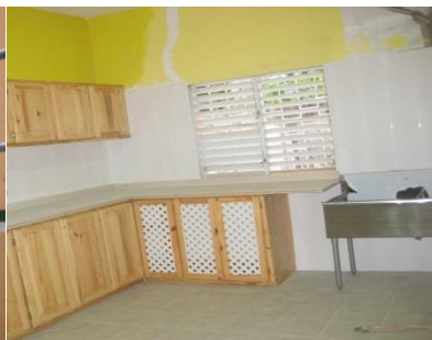
Kitchen cupboards and kitchen sink installed
