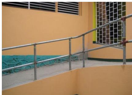
Metal grill work, painting, ramp for the disabled with handrails
