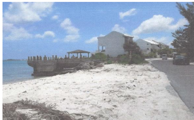
The eastern portion of the work site at Sandyport Beach
