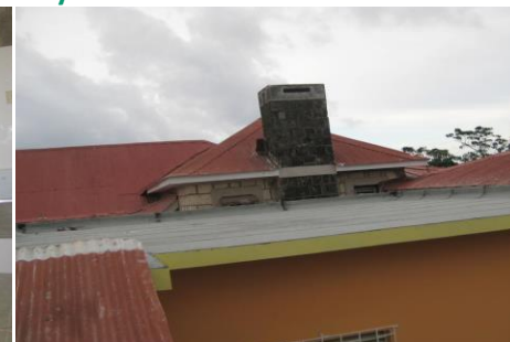
Waterproofing Membrane installed on roof slab
