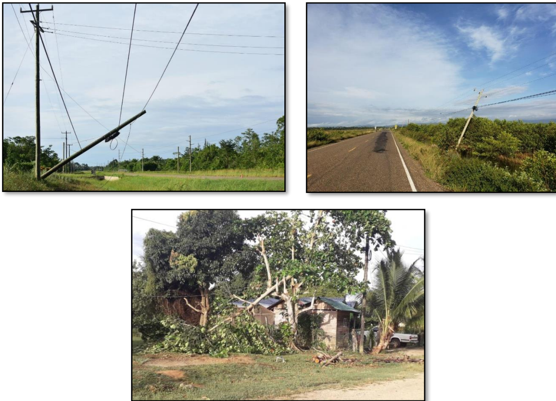
Figure 5 Some of the wind damage caused by Hurricane Nana in Belize – September, 2020. Source: Belize Electricity Limited and News 5 Live
