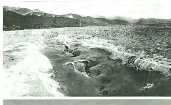
Figure 12: Liquefaction and Foundation Failure in Harbour View and Port Royal in 1907 Earthquake Area close to Harbour View end of Palisadoes (Adopted from Ahmad 2011)
