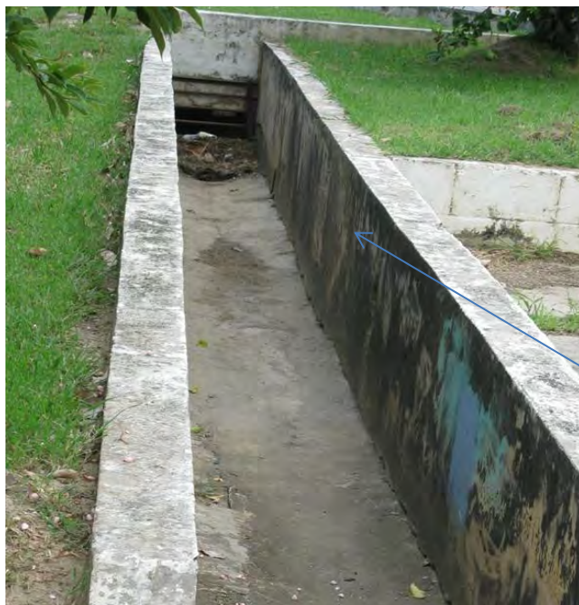
Photograph 4.18 Inadequate drainage to remove flood waters
