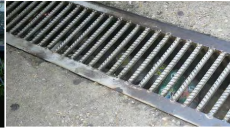
Photograph 4.8 Storm drain filled with garbage
