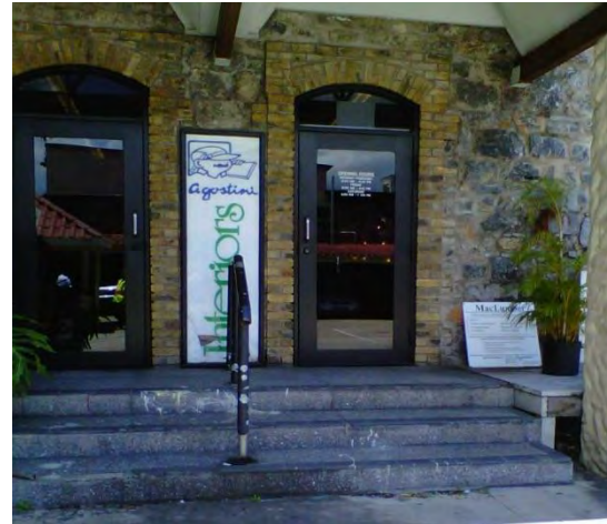
Photograph 4.13. Business raised floors to prevent water from entering
