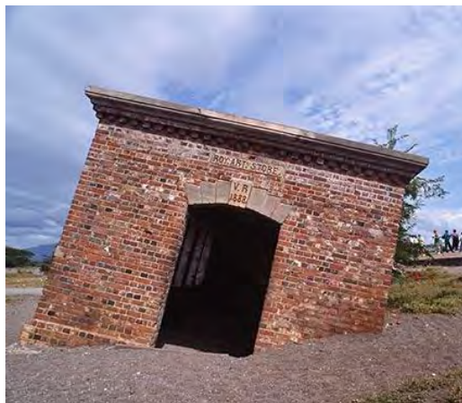
Figure 13: Old Artillery House/ Giddy house in Port Royal that suffered foundation failure in 1907 (Ahmad , 2011)
