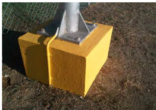
Figure 19: Photograph showing type of utility pole at NMIA Facility (Photograph K.Douglas)
