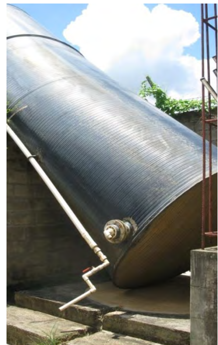
Photograph 4.17 Empty water tank which was toppled by the force of flood waters in June 2011 flood
