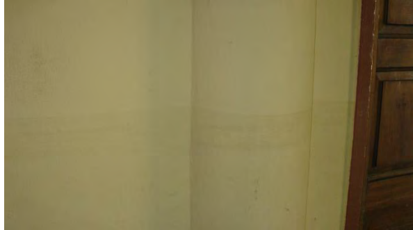
Photograph 4.15 Flood water mark of flood event in 2003
