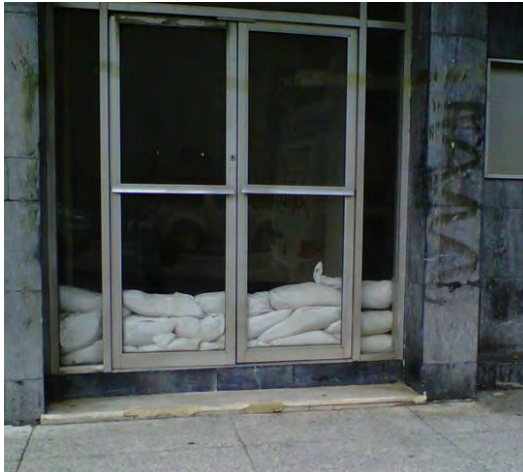
Photograph 4.11 Sandbags positioned at doorway at business on St. Vincent Street, Port of Spain
