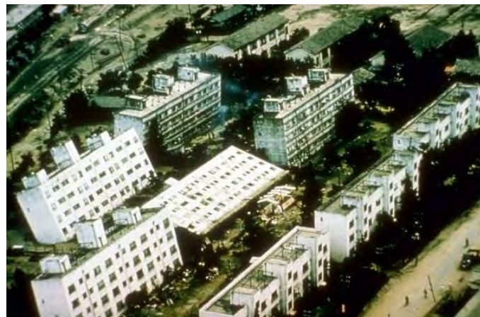
Figure 14: Photograph showing earthquake-resistant buildings affected by Liquefaction in Niigata, Japan- June 16, 1964 ( www.USGS.gov.earthquakes )
