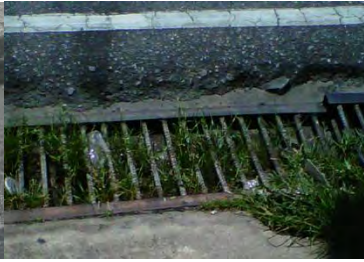
Photograph 4.7 Overgrown storm drain grate
