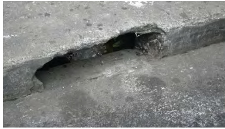
Photograph 4.6 Storm drain filled with garbage
