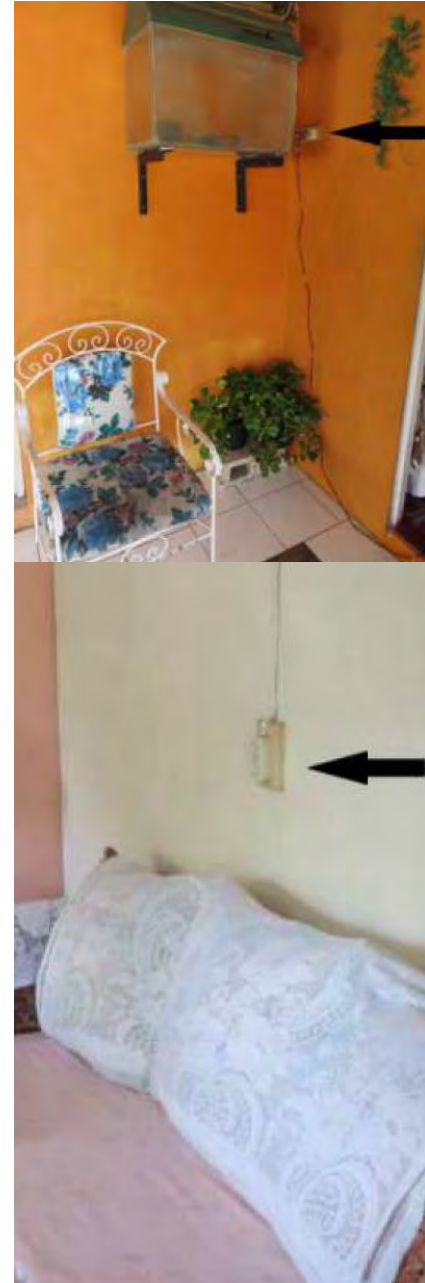
Figure 6: electronic fixtures above the usual height of flood waters
