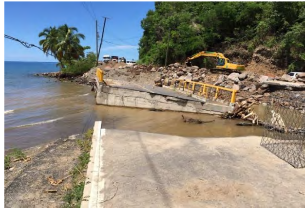
Picture of collapsed bridge due to Tropical Storm Erika floods at Coulibistrie
