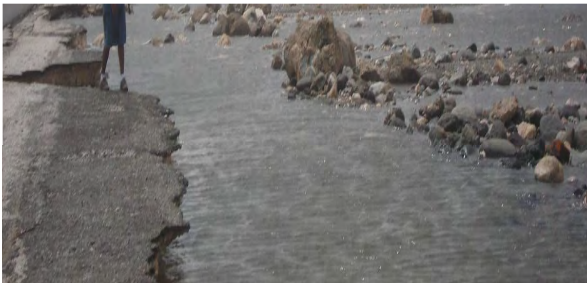
Figure 16: Photograph showing section of NMIA Roadway damaged during Hurricane Dean Adapted from Marine Geology Unit, UWI 2007
