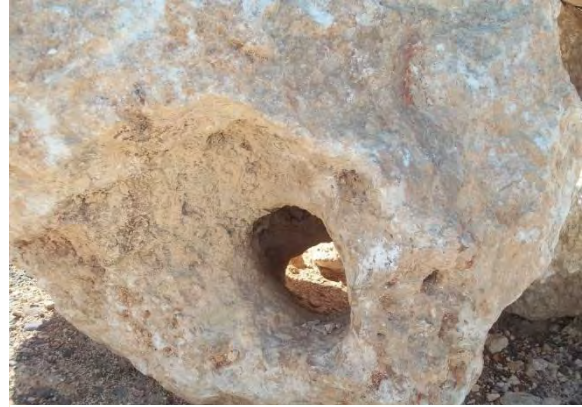
Fig. 17: Photograph showing a limestone boulder used as revetment along Palisadoes Road – showing Areas of weakness which can be chemically weathered over time
