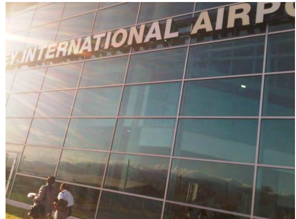
Figure 20: Photograph showing large glass section of new terminal building at NMIA (Photograph by K. Douglas)
