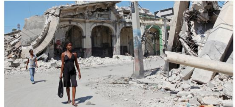
Devastation caused by the 2010 Haiti Earthquake
