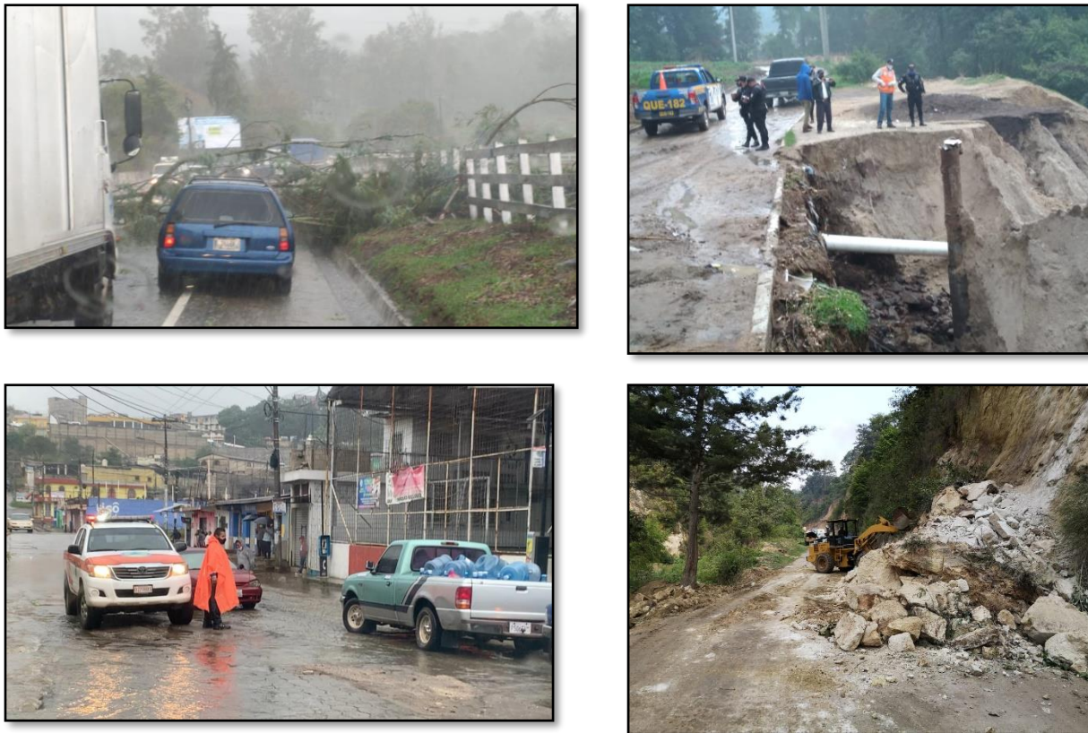
Figure 4 Damage caused by this adverse weather period in Guatemala – May 2020 Source: Coordinadora Nacional para la Reducción de Desastres
