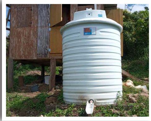
Photo 4: Tanks used for rainwater harvesting in Grenada
