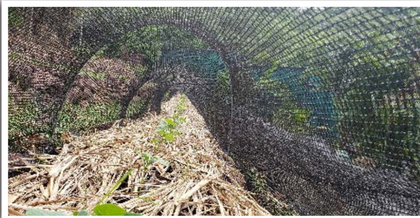
Photo 17: Galvanized steel rod arch.
