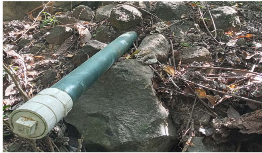
Photo 5: Buried pipe at natural spring site
