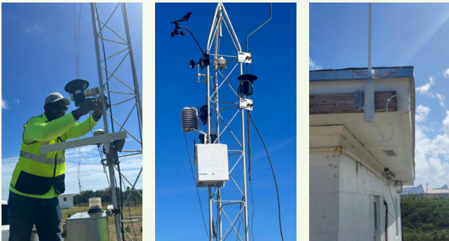
Installations of the CCRIF-funded Automated Weather Systems at the Grand Turk airport and the South Caicos airport
