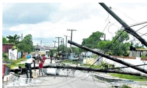
Damage in Jamaica caused by Hurricane Sandy
