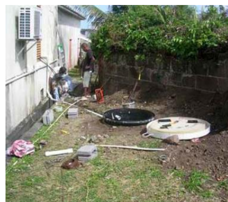
Installation of Strong Motion Station behind the disaster office at Fort Frederic, Grenada
