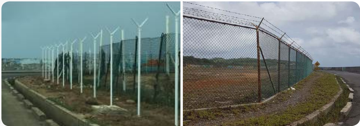
The new fencing at Douglas-Charles Airport in Dominica
