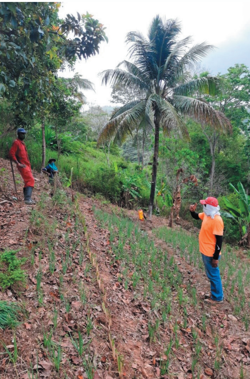
Installing vetiver grass to stabilize this hillside and protect against soil erosion and improve the quality of the soil
