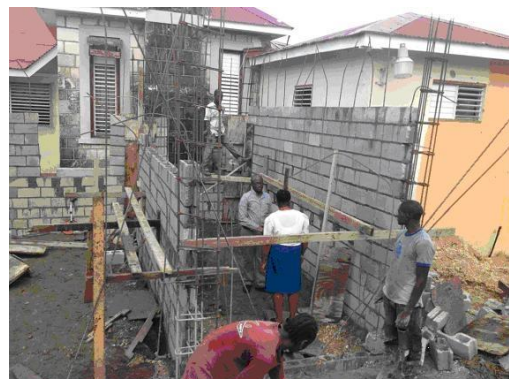
Construction of the new kitchen at Muirton Boys Home
