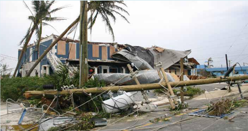
Damage resulting from Hurricane Ivan's impact on Cayman in September 2004
