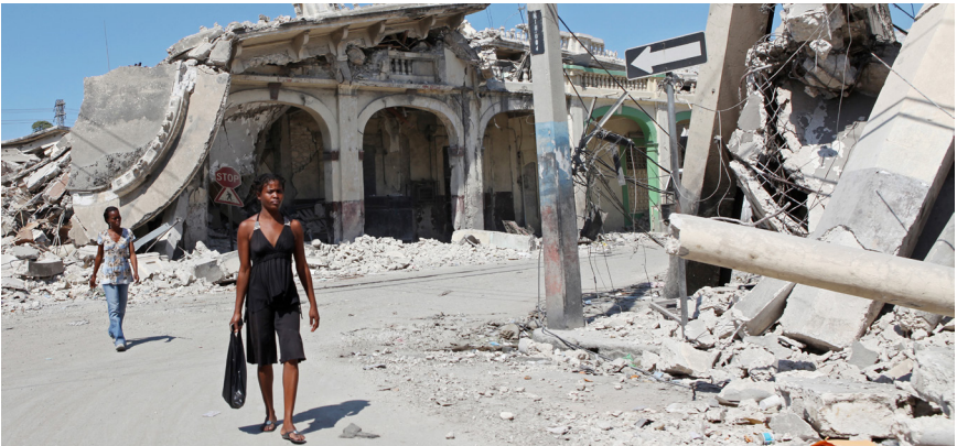
Devastation caused by the 2010 Haiti Earthquake
