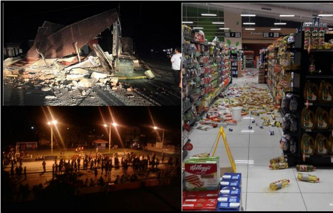
Figure 2 Damage caused by the earthquake on 10 June 2016 in Nicaragua. Source: El Nuevo diario and 100 noticias.
