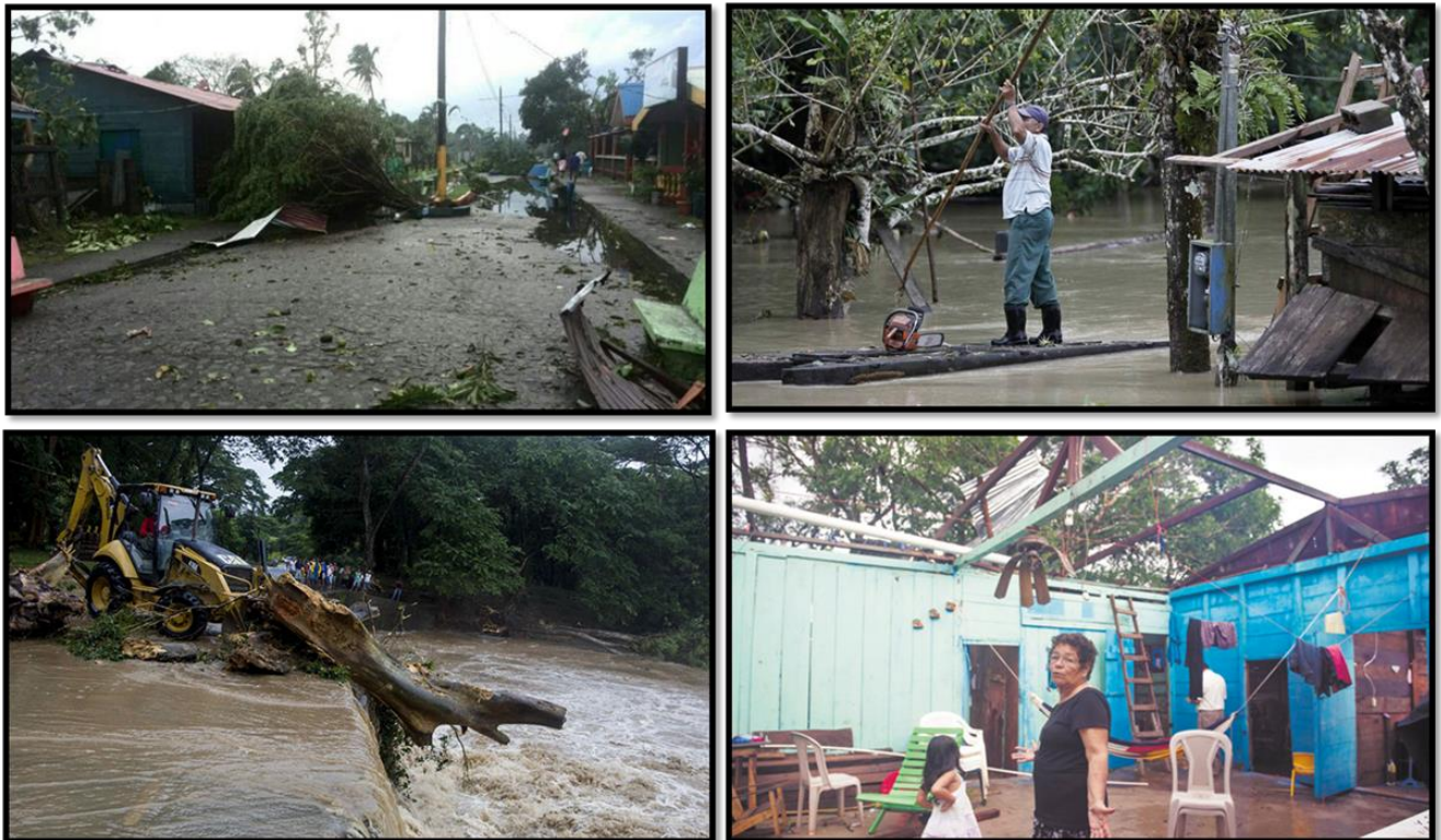
Figure 6 Desolation and destruction after Hurricane Otto in Nicaragua. Source: El Nuevo Diario - Nicaragua
