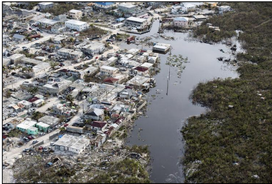
Figure 5 Damage caused by Hurricane Irma in the Turks and Caicos Islands – September 2017.
