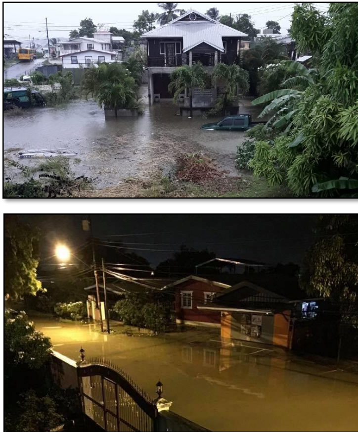
Figure 6 Damage caused by heavy rainfall in Barbados – September 2018. Sources: Magnetic Media and Loop
