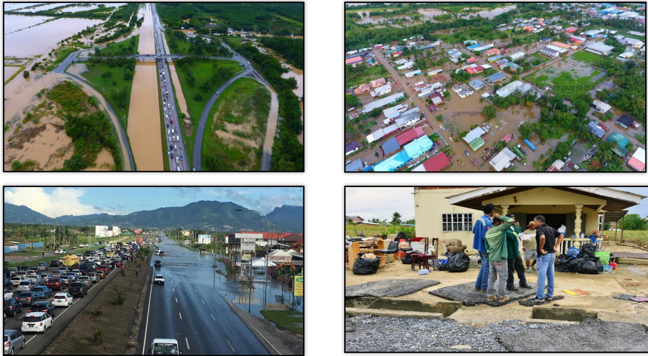
Figure 5 Damage caused by heavy rainfall in Trinidad – October 2018. Sources: Trinidad Express Newspapers, Loop and Jamaica Observer
