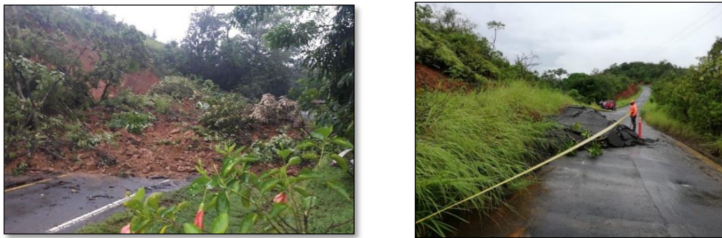
Figure 3 Damage caused by this adverse weather period in Panama – August 13-21, 2020 Source: Sistema Nacional de Protección Civil
