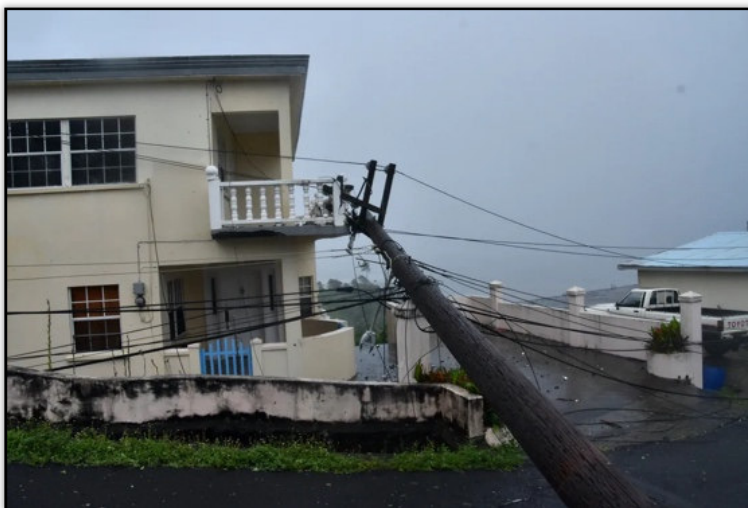
Figure 8 Some damage caused by Tropical Storm Elsa in St. Vincent and The Grenadines – July 2021. Source: CBC Radio-Canada
