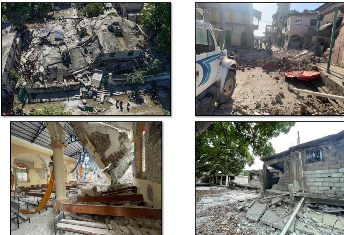
Figure 9 Damage caused due to M7.2 earthquake in Haiti. August 2021. Source: The New York Times, OCHA, Enfield Independent and Miyamoto International
