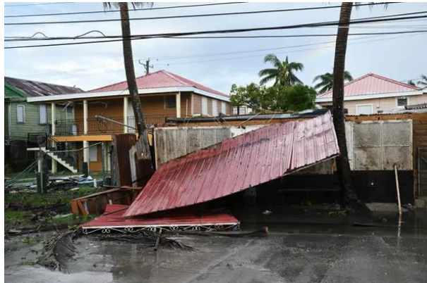
d) Fallen roof tops
