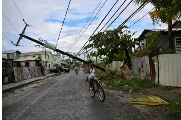
b) Utility poles fallen down
