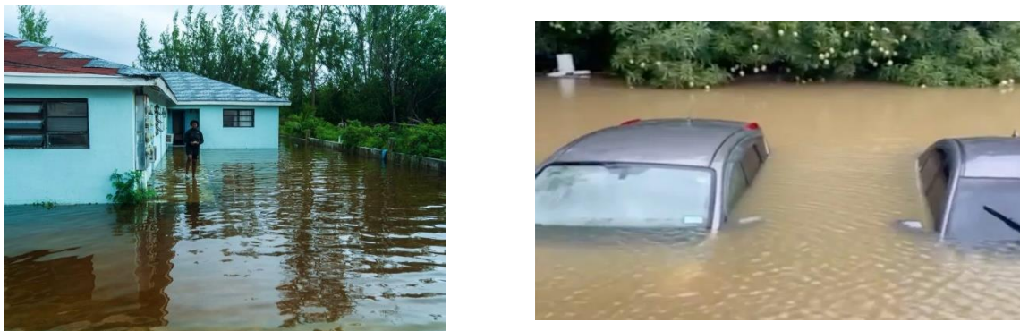
Figure 3 Flood damage in Exuma
