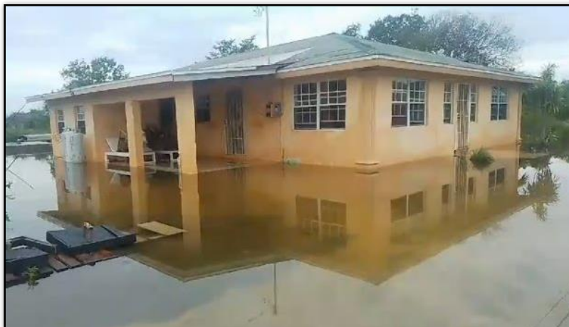
Figure 4 Flooding damage in Matthew Town, Inagua
