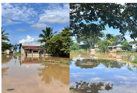
b) Flooding and Damage Assessment and Needs Analysis Los Angeles, Chisec, Alta Verapaz 7
