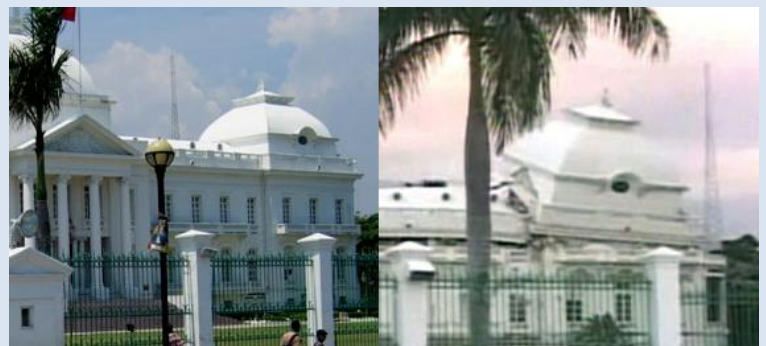
The Presidential Palace before and after the earthquake
