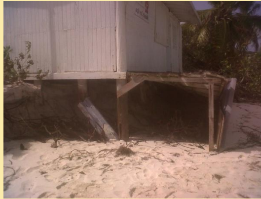
Photo at left shows clean-up activity in Anguilla following Hurricane Earl. Photo at right shows an undermined building at Shoal Park east in Anguilla
