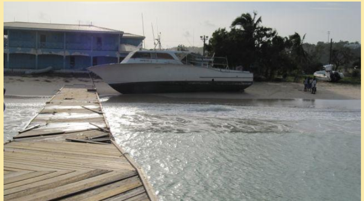
Damage to police jetty in Anguilla as a result of the passage of Hurricane Earl
