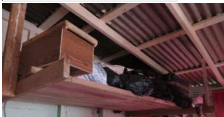
Figure 5: Furniture constructed to protect household items in future floods*
