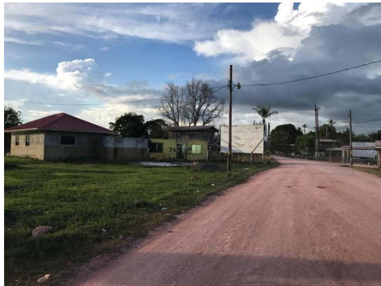
Figure 5.9 Road development usually affected by floods in Kwakwani
