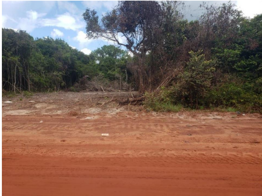
Figure 5.3 Land clearing for housing construction.
