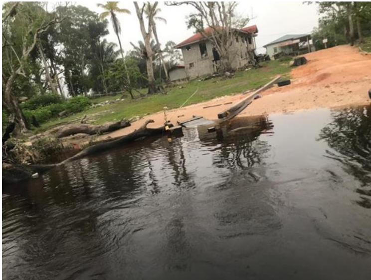
Figure 5.6 Housing development in the Kwakwani floodplain
