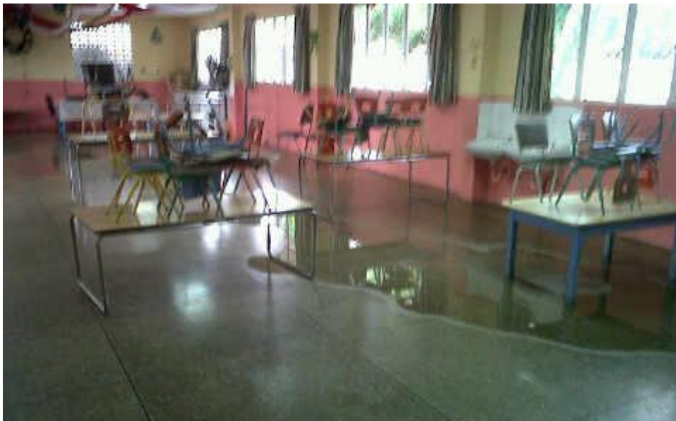
Photographs 2.4 and 2.5 Showing Flooding on November 19 th 2011 at Princess Elizabeth Centre
