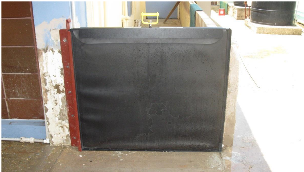
Photograph 4.20 Flood barrier placed at entrance to Orthopaedic surgery theatre to prevent flood waters from entering
