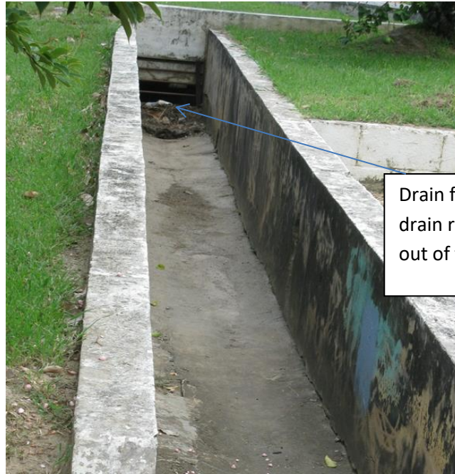
Photograph 4.18 Inadequate drainage to remove flood waters
