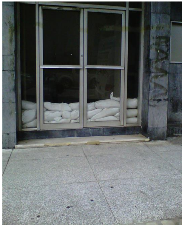
Photograph 4.11 Sandbags positioned at doorway at business on St. Vincent Street, Port-of-Spain
