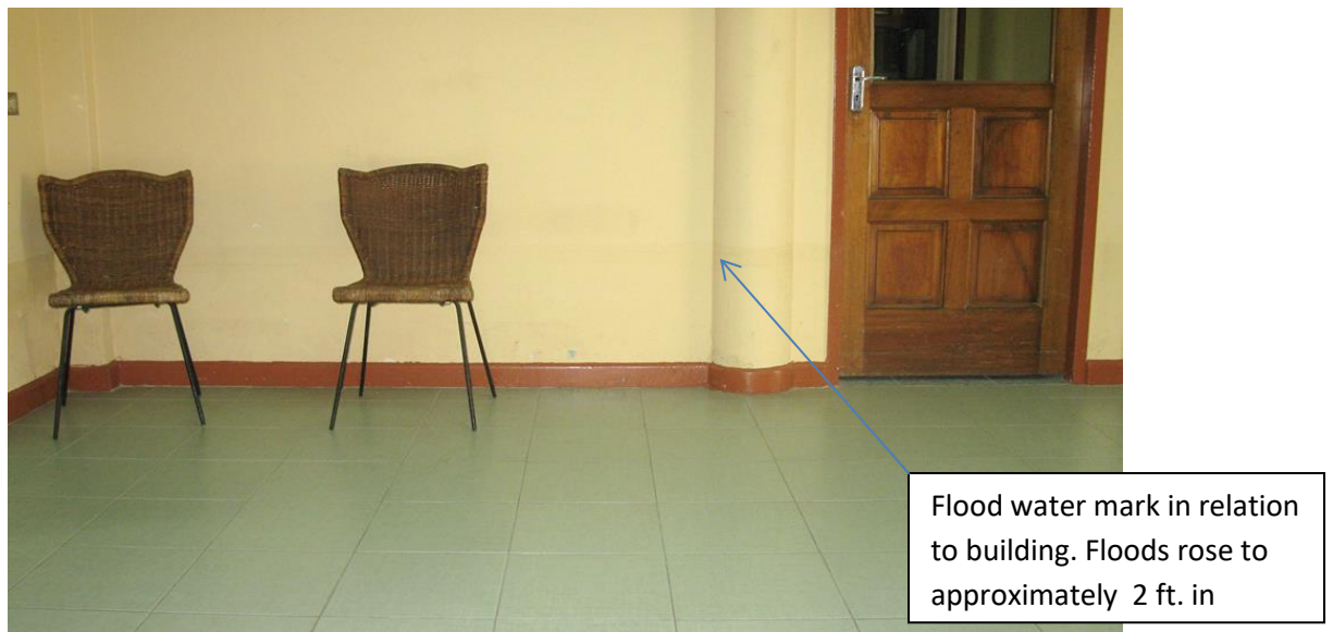
Photograph 4.16 Illustrates the height of the flood in relation to the surroundings, showing the flood to be approximately two feet in some places.
