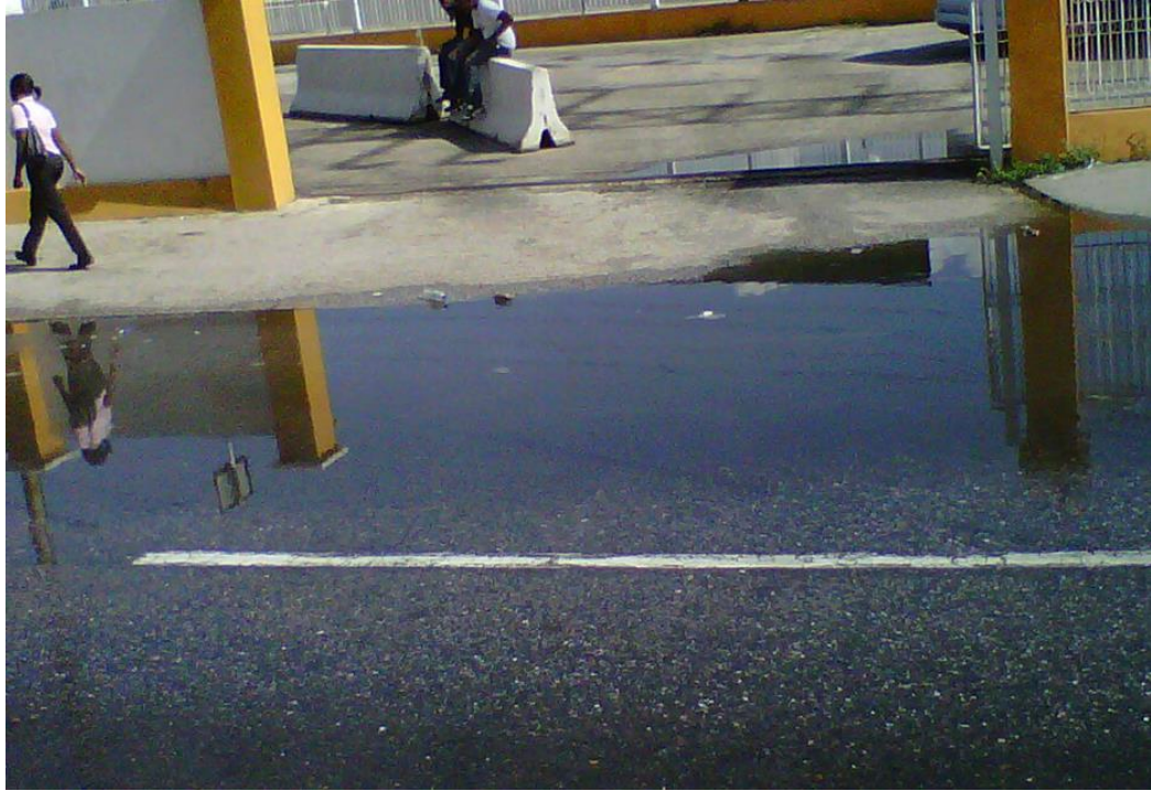
Photograph 4.5 Ponding of water along road way after short rainfall
