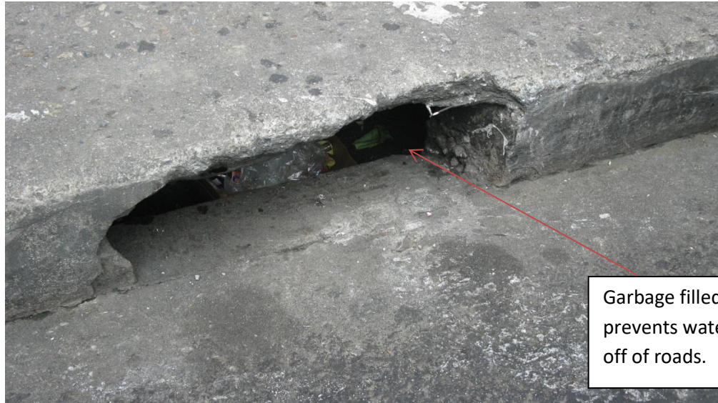
Photograph 4.6 Storm drain filled with garbage
