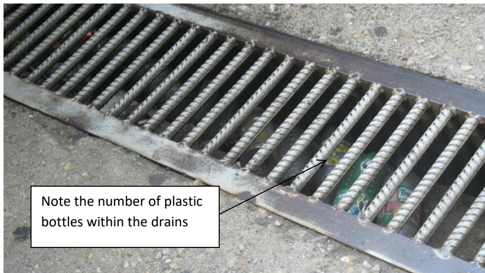
Photograph 4.8 Storm drain filled with garbage
