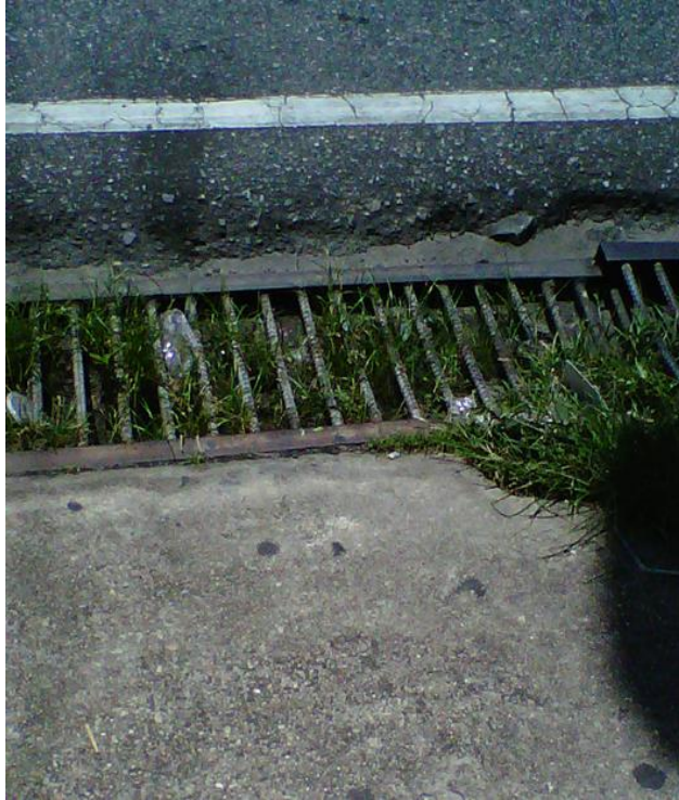
Photograph 4.7 Overgrown storm drain grate
