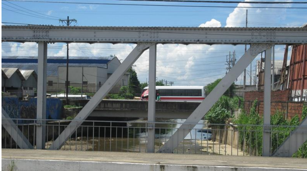
Photograph 4.10 Seaward view of East Dry River. Note the presence of buildings on either side of the river channel as well as low bridges across the waterways.
