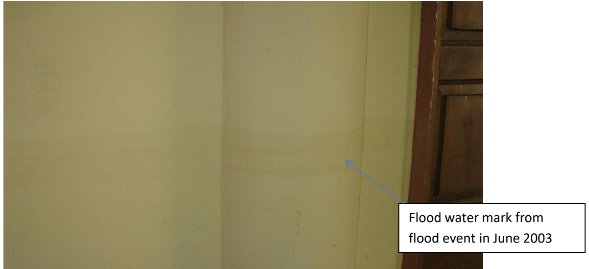
Photograph 4.15 Flood water mark of flood event in 2003
