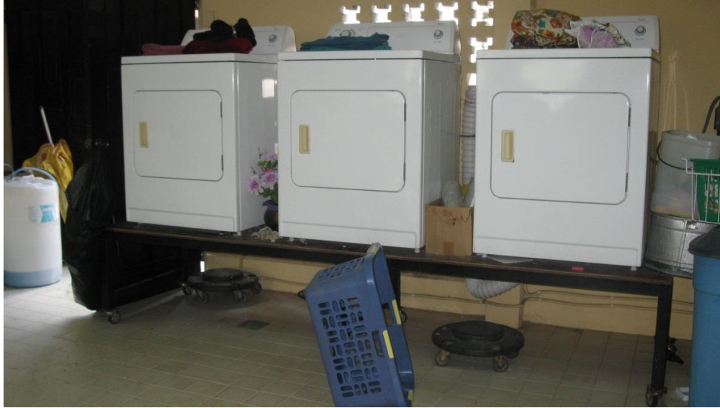
Photograph 4.19 Measures taken to reduce the impact of flood events
