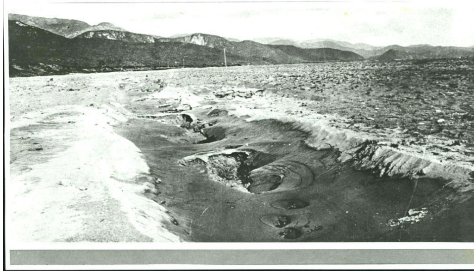
Fig.11- Liquefaction and Foundation Failure in Harbour View and Port Royal in 1907 Earthquake
