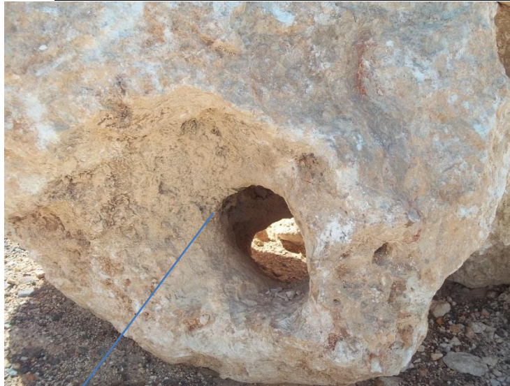
Fig. 17: Photograph showing a Limestone Boulder used as revetment along Palisadoes Road (Photograph K. Douglas)
