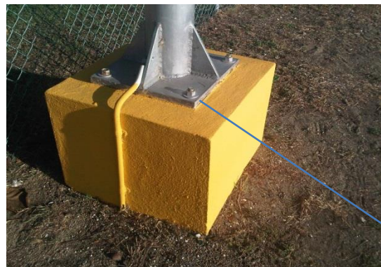
Figure 19: Photograph showing type of utility pole at NMIA Facility (K.Douglas Photograph)
