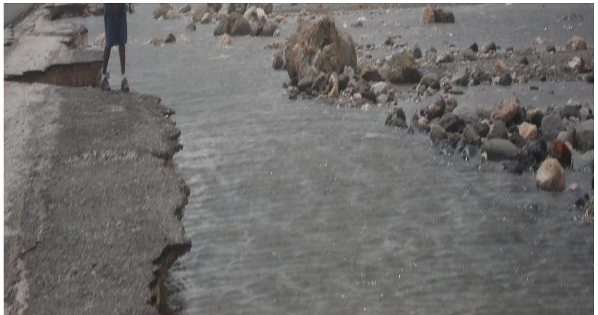
Fig 16: Photograph showing section of NMIA Roadway damaged during Hurricane Dean
