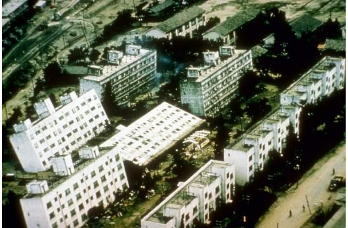
Fig.14- Photograph showing earthquake resistant buildings affected by Liquefaction in Niigata, Japan- June 16, 1964
