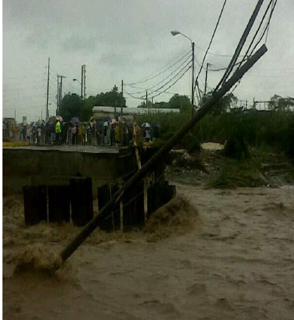
Figure 11 Damaged Bridge. Source: Weather.
