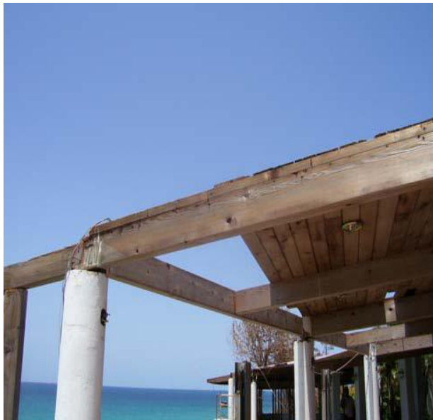
Figure 5 Example of damage to a hotel. Source: CIMH.
