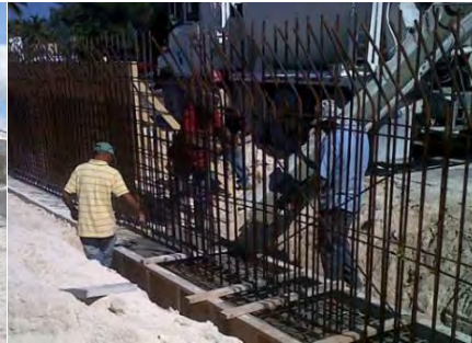
Construction of the sea wall
