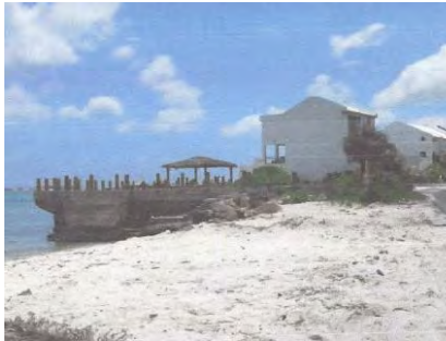
Sandy Port Beach in The Bahamas before work began
