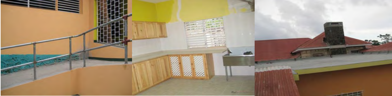
Metal grill work, painting, ramp for the disabled with handrails
