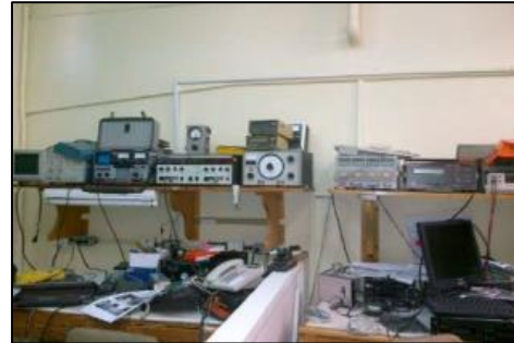
Plates 9 and 10: Loose electrical wiring at work stations
