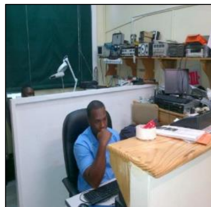
Plates 5 and 6: Earthquake equipment poorly stored above occupied cubicle stations.
