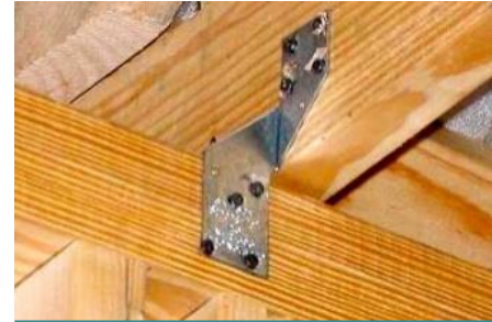
A hurricane strap provides extra support for a roof
